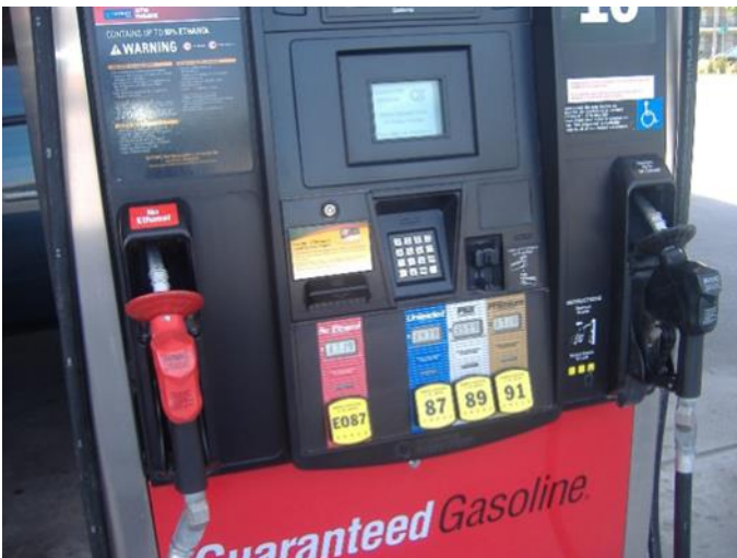
E087 Button marked, No Ethanol. Also, pump handle is red.
